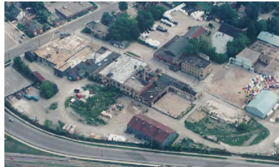
Canbar operation prior to demolition
