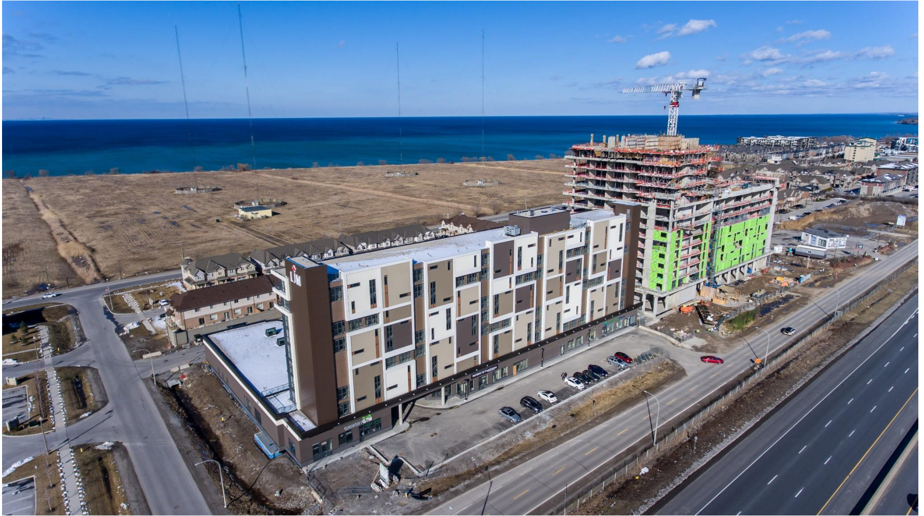
Image 6: 565 North Service Road, Grimsby ON – internal view – away from noise source
