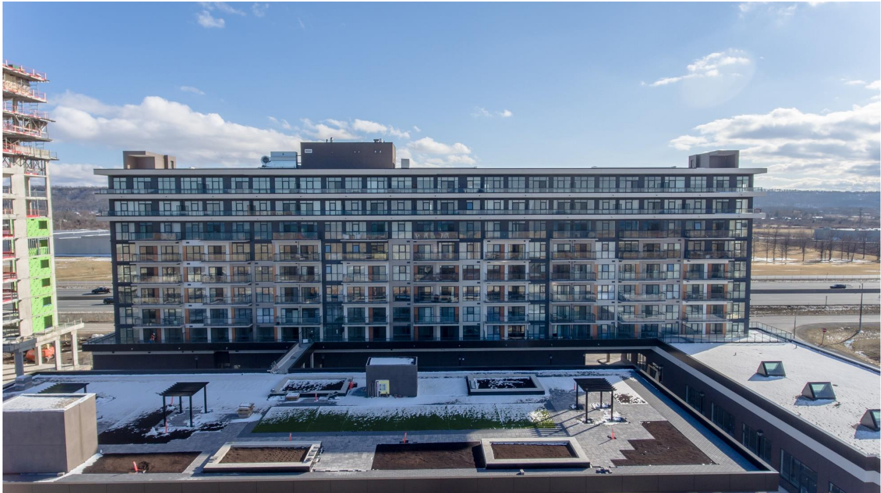
Image 5: 565 North Service Road, Grimsby ON – internal view – away from noise source
