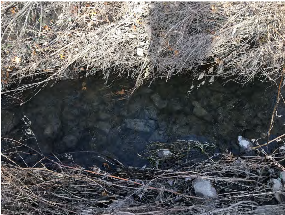
Photo 10: Angular stone substrate within the Conrail drain within the TWGC (November 2017).
