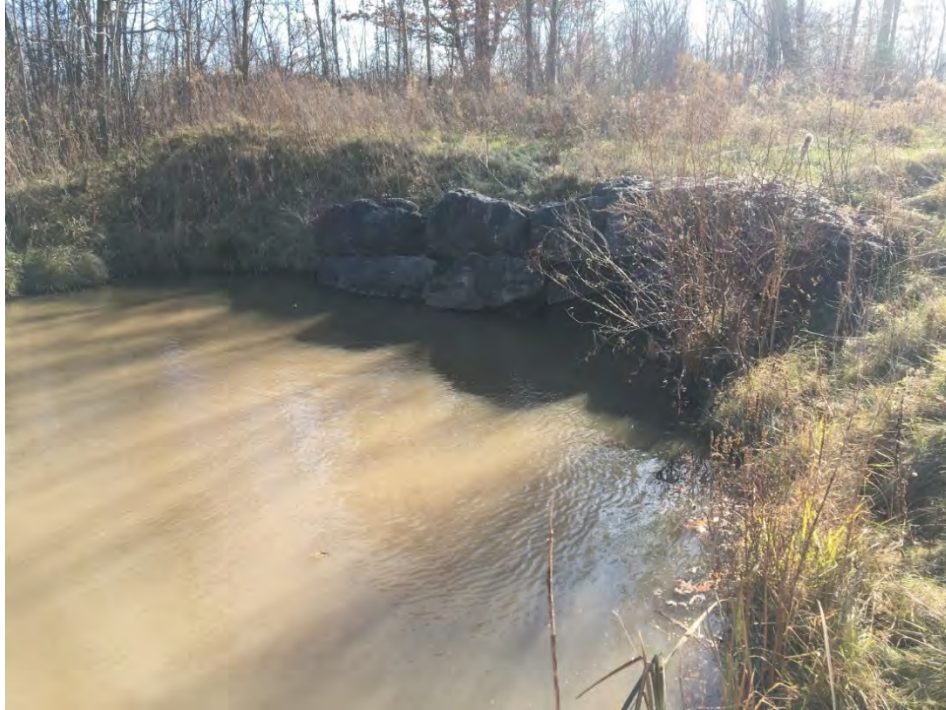
Photo 12: Looking South, Pond E within the Thundering Waters Golf Course property (November 2017).
