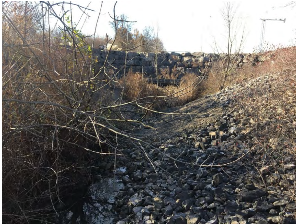
Photo 5: Looking southwest at the concrete siphon culvert through which the Conrail Drain flows, upstream of John Daly Way (November, 2017).
