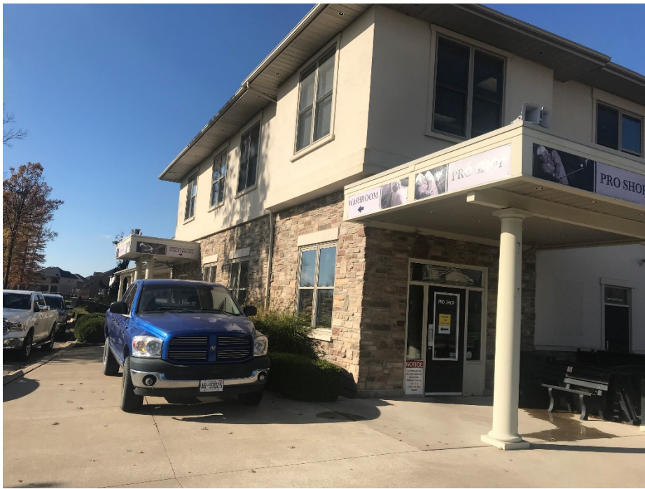
Photograph 1: General view of main clubhouse building.
