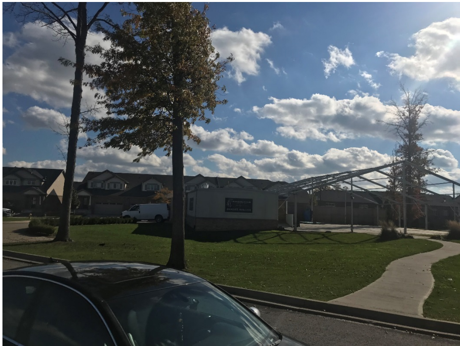
Photograph 2: General view of catering building.
