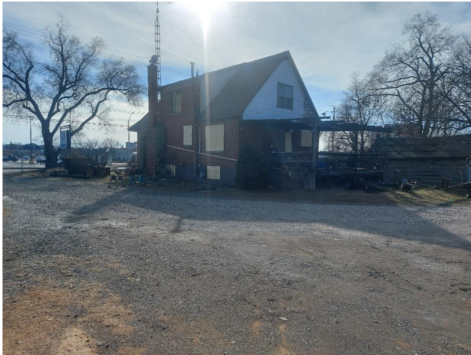
Image 2: Study Area Conditions. Facing South.
