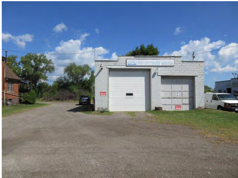
PHOTOGRAPH 2: VIEW OF VACANT COMMERCIAL BUILDING ONSITE
